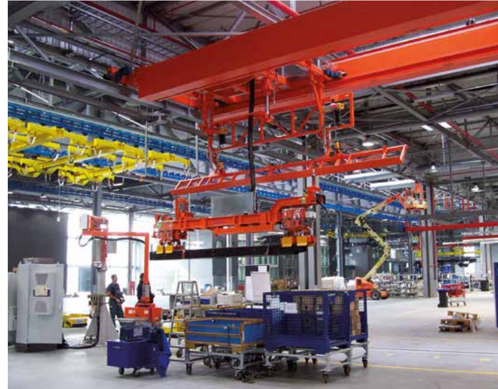
Assembly crane, zig-zag solution
